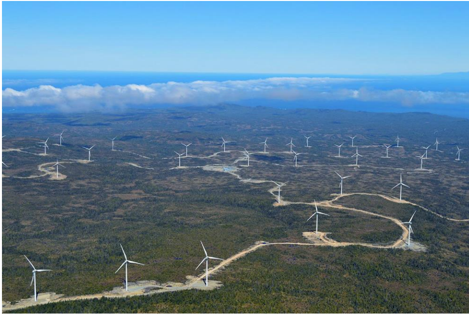
The Cape Scott Wind Farm produces clean energy for Vancouver Island communities and industries, yet when the North Island has power outages, local communities cannot access this local supply of clean electricity.
