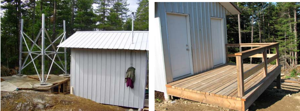
The GBIS building on Pocahontas contains routers and the PEP emergency repeater equipment.
