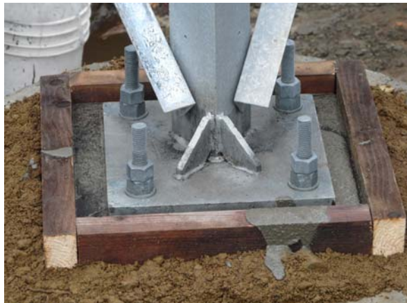
Over 200 bags of special concrete were used on the base, plus special grout on each leg.
