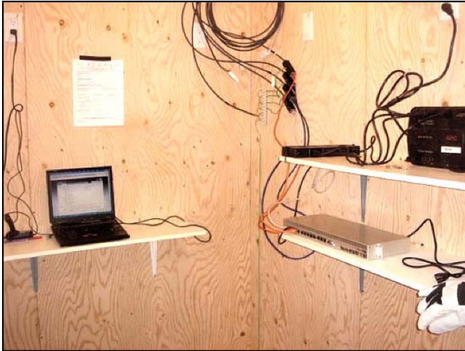
Equipment in the GBIS building on Pocahontas; on the right is the PEP emergency repeater equipment.
