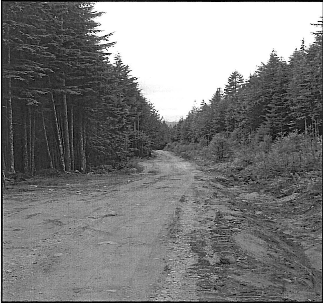
Picture 2: Road Construction After Stage 1; Right of Way Clearing
