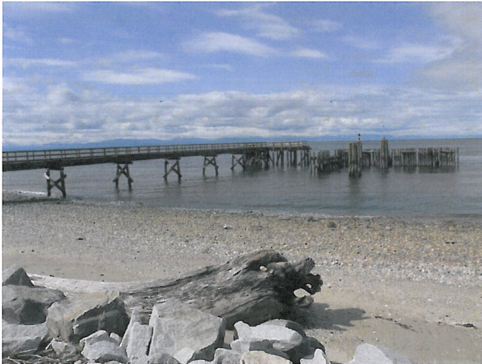
Davis Bay Wharf – Prior to 2014 Construction
