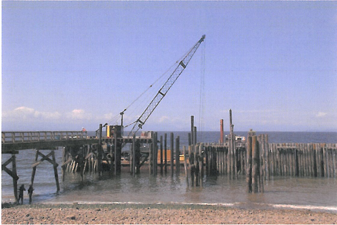
Davis Bay Wharf – During 2014 Construction
