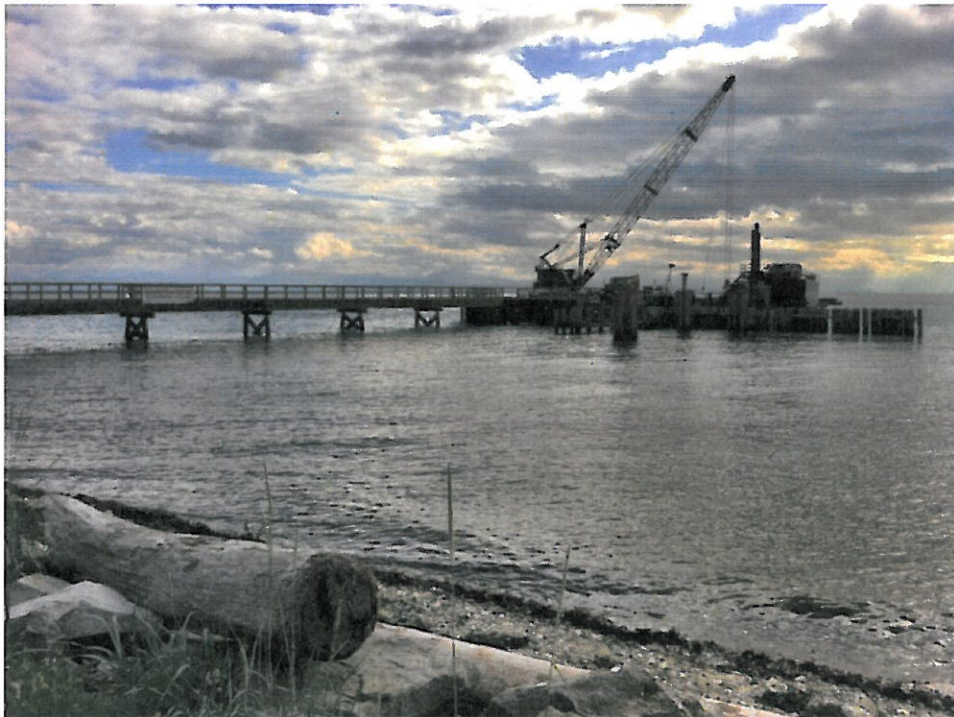
Davis Bay Wharf – During 2014 Construction
