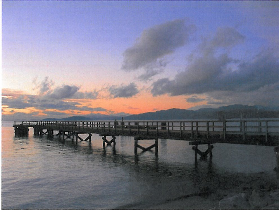
Davis Bay Wharf – Prior to 2014 Construction
