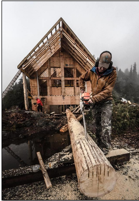
Image 7: Preparing the hut's front centre post for installation.
