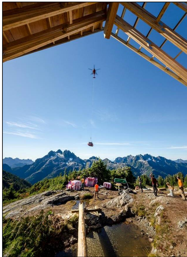
Image 4: Helicopter dropping off more supplies during the build (September, 2017).
