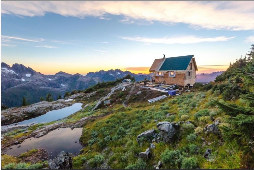
Image 5: South side of the hut during the build (September, 2017).
