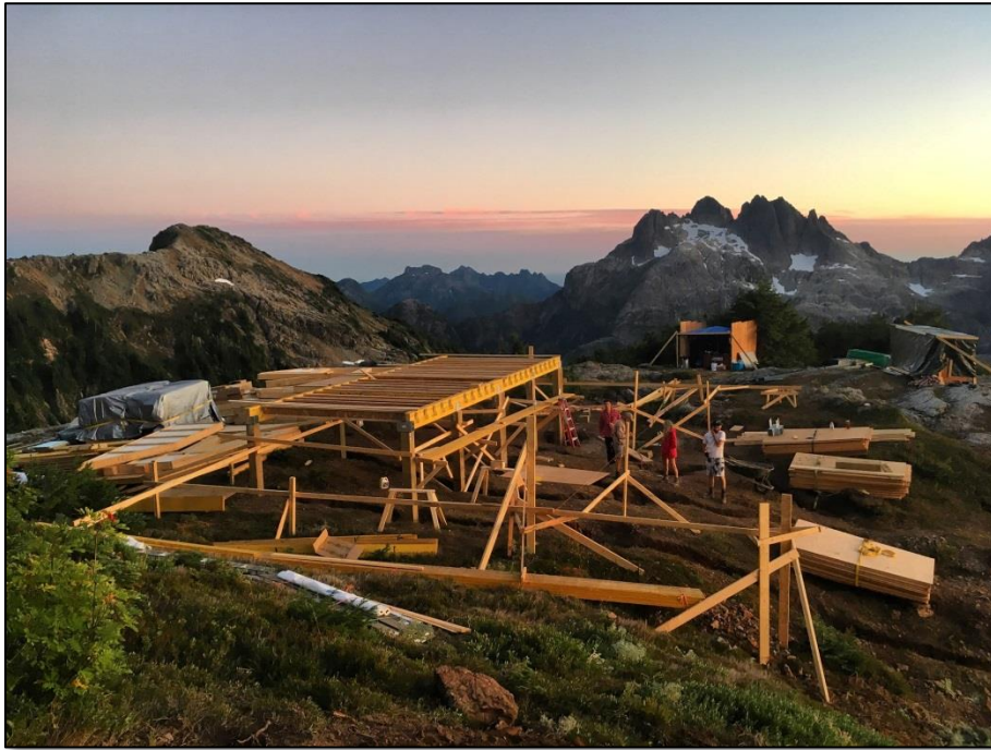
Image 3: Early construction on the hut's foundation (August, 2017).
