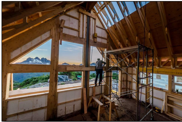
Views from inside the hut when construction was 50% complete.
