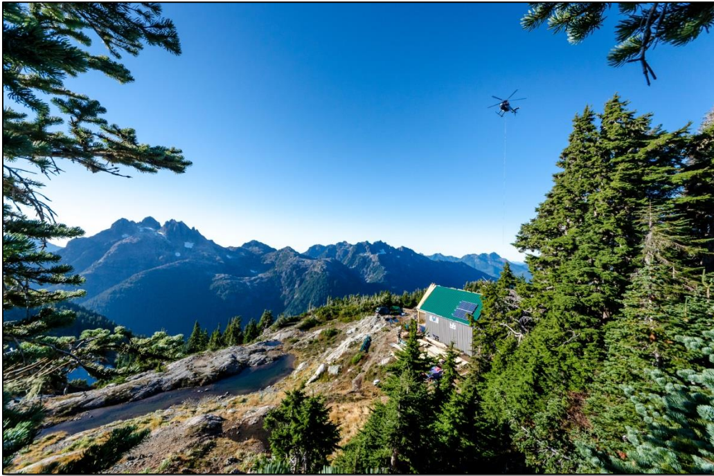
Image 9: The weather tight hut at the end of the 2017 construction, October 28, 2017.
